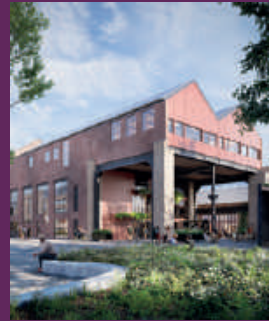
PATTERN SHOP OFFICE BUILDING
