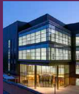
ROCKET OFFICE BUILDING
