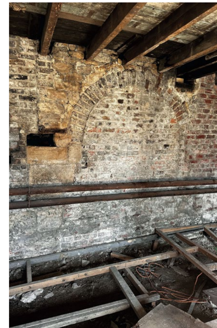
Machine Shop, details to be retained
