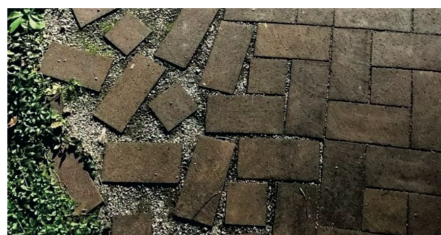
Reclaimed materials : brick paving
