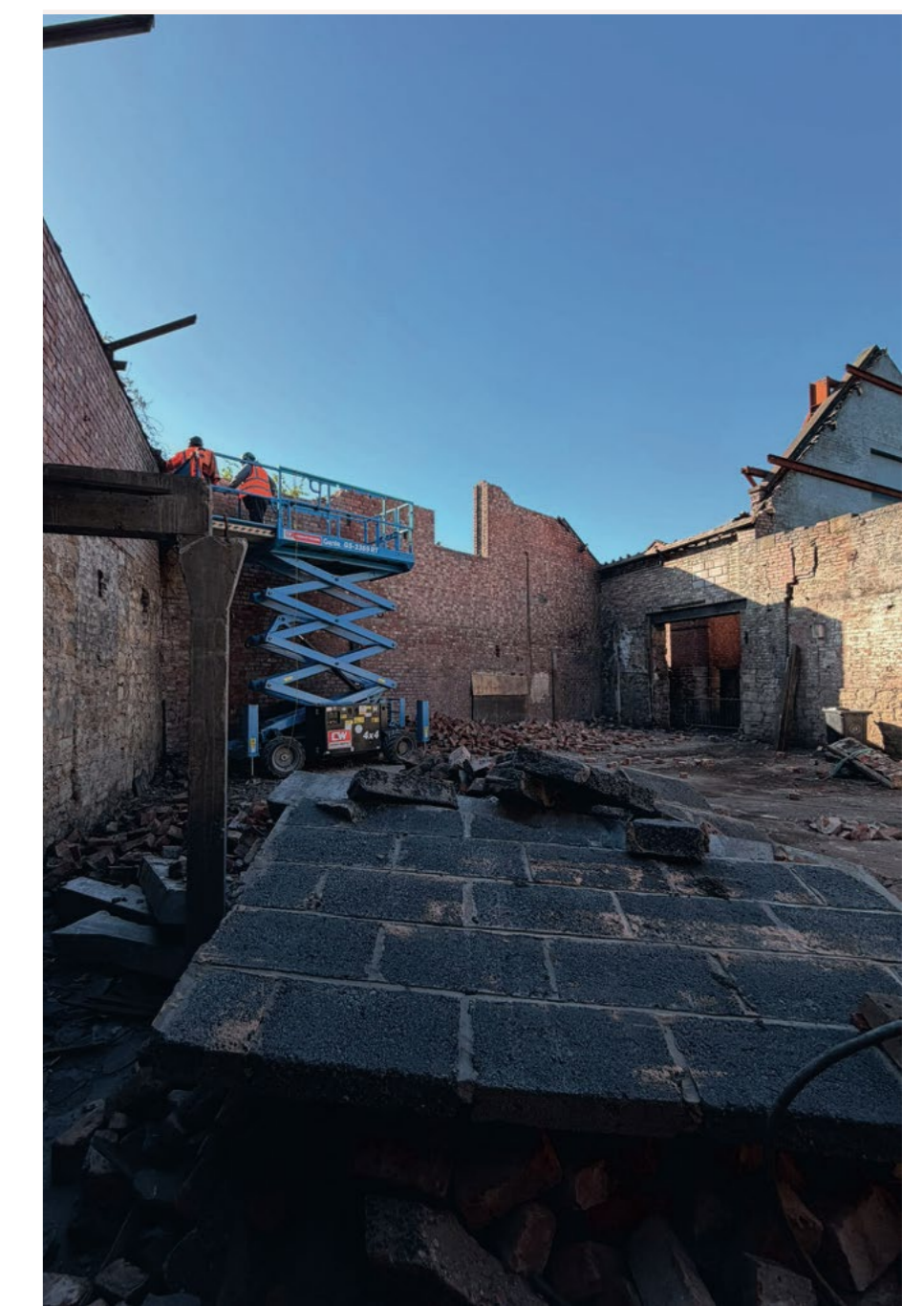
Machine Shop, demolition of modern fabric
