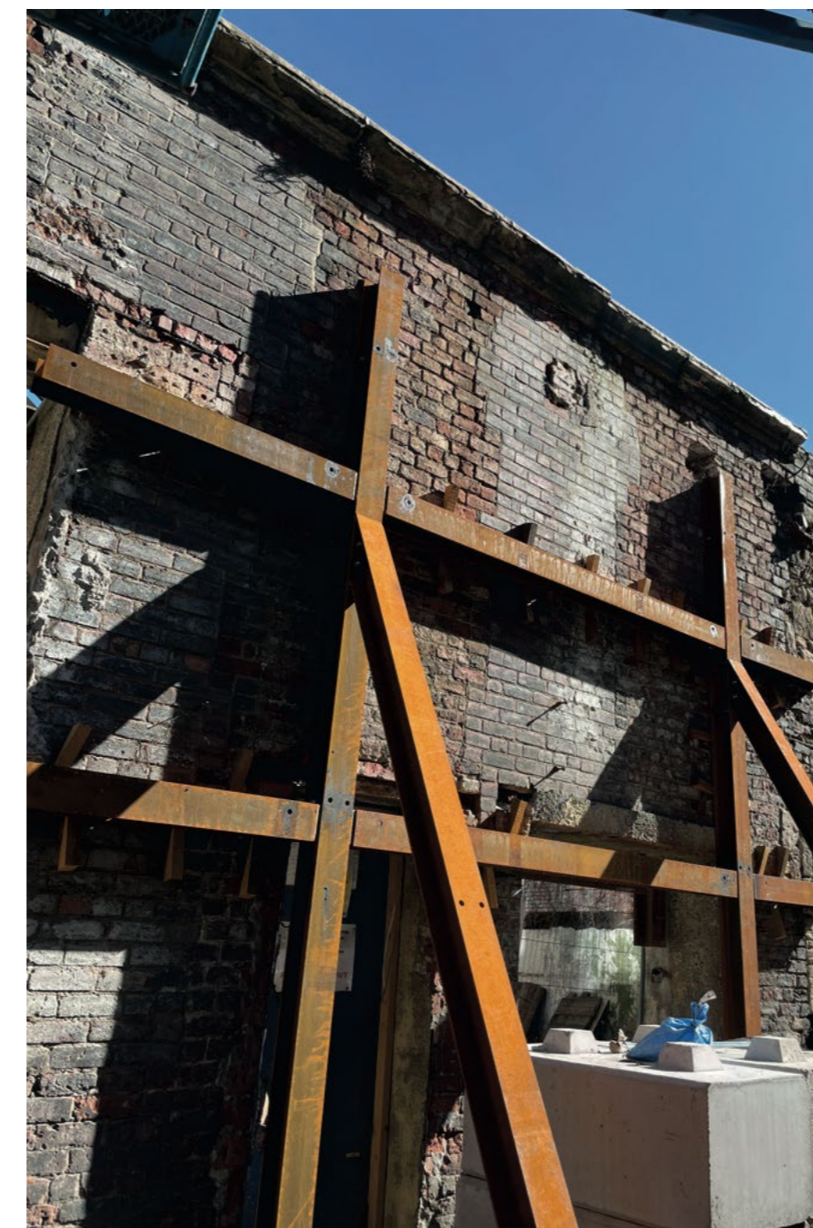
Temporary support of heritage fabric
