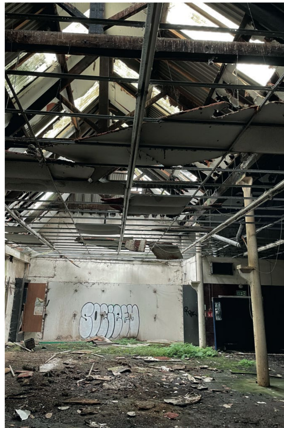
Machine Shop, before strip out
