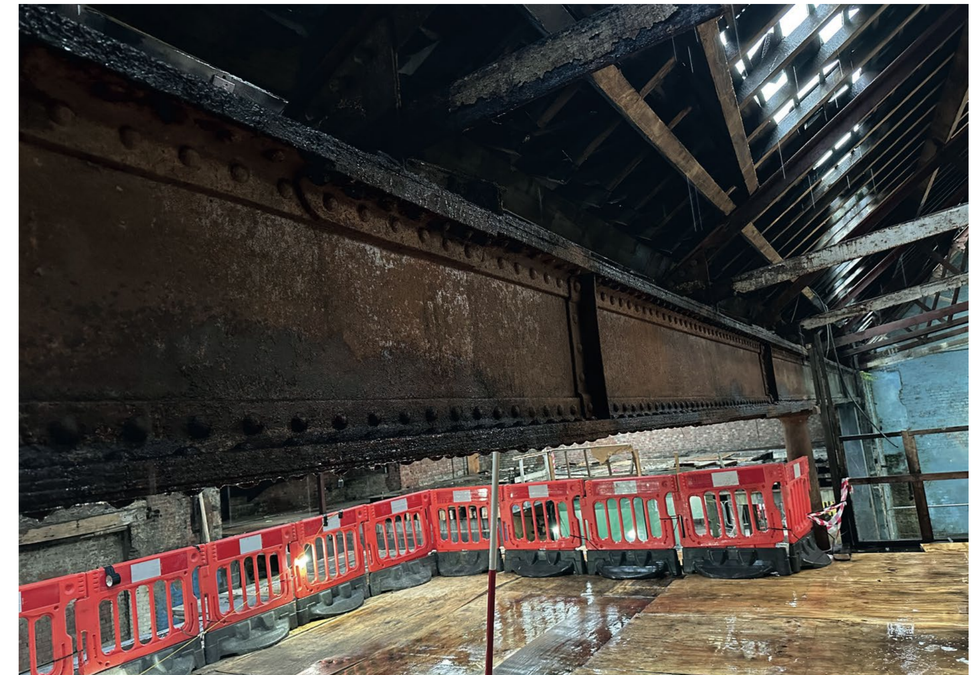
Machine Shop, details to be retained
