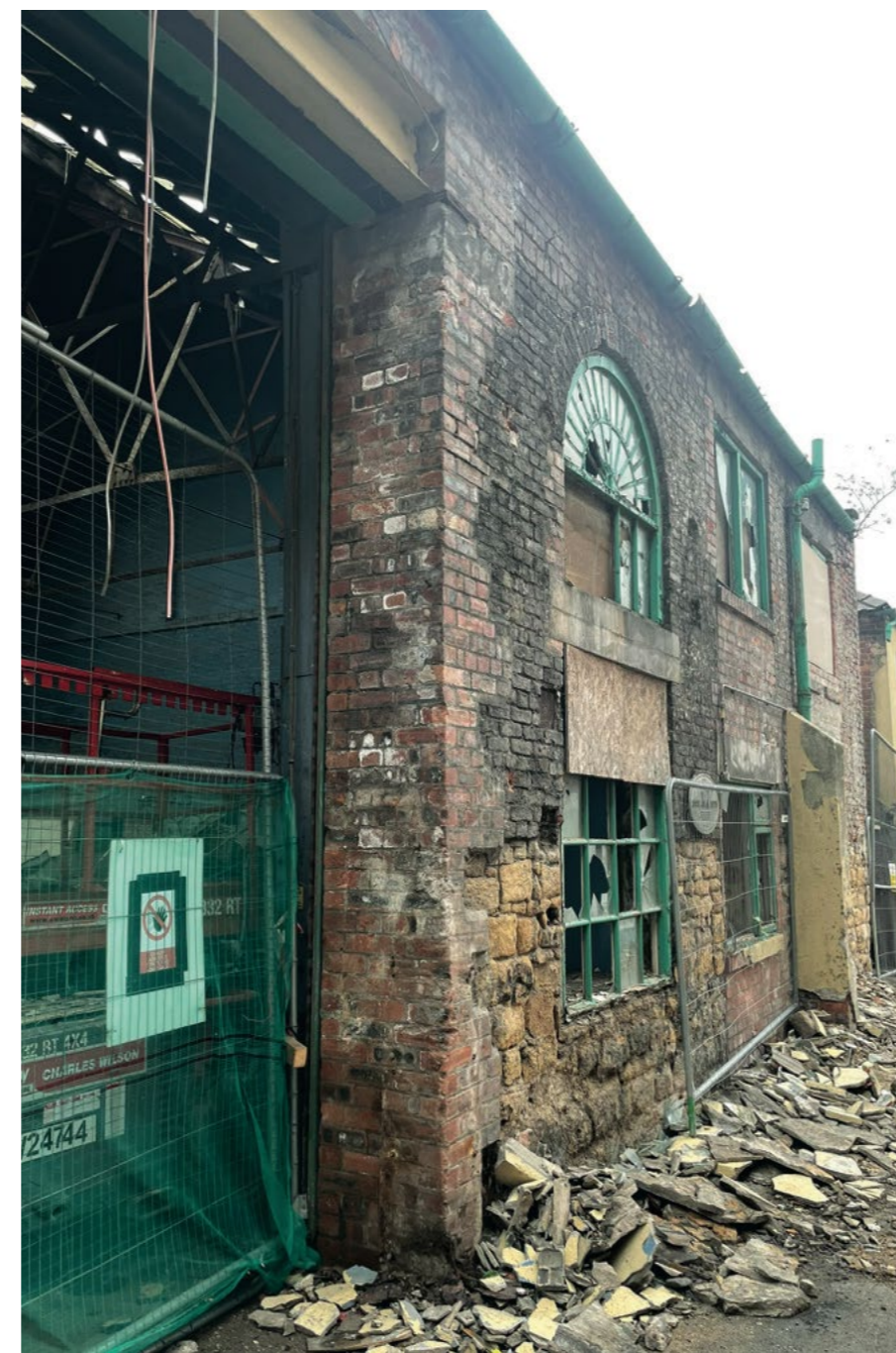
South Street wall, after render removal
