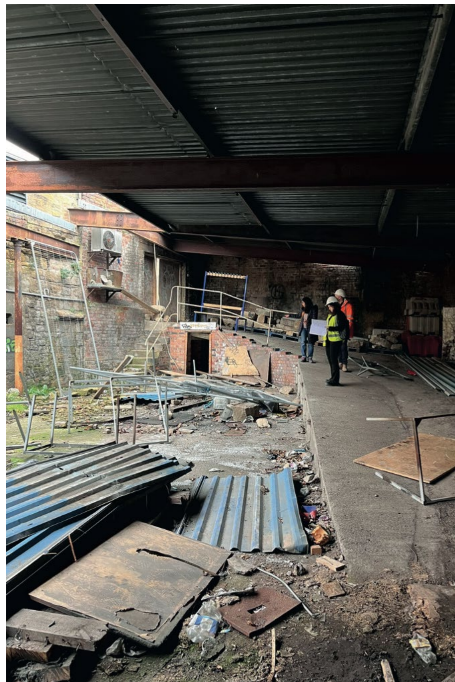
Smith Shop, before removal of roof
