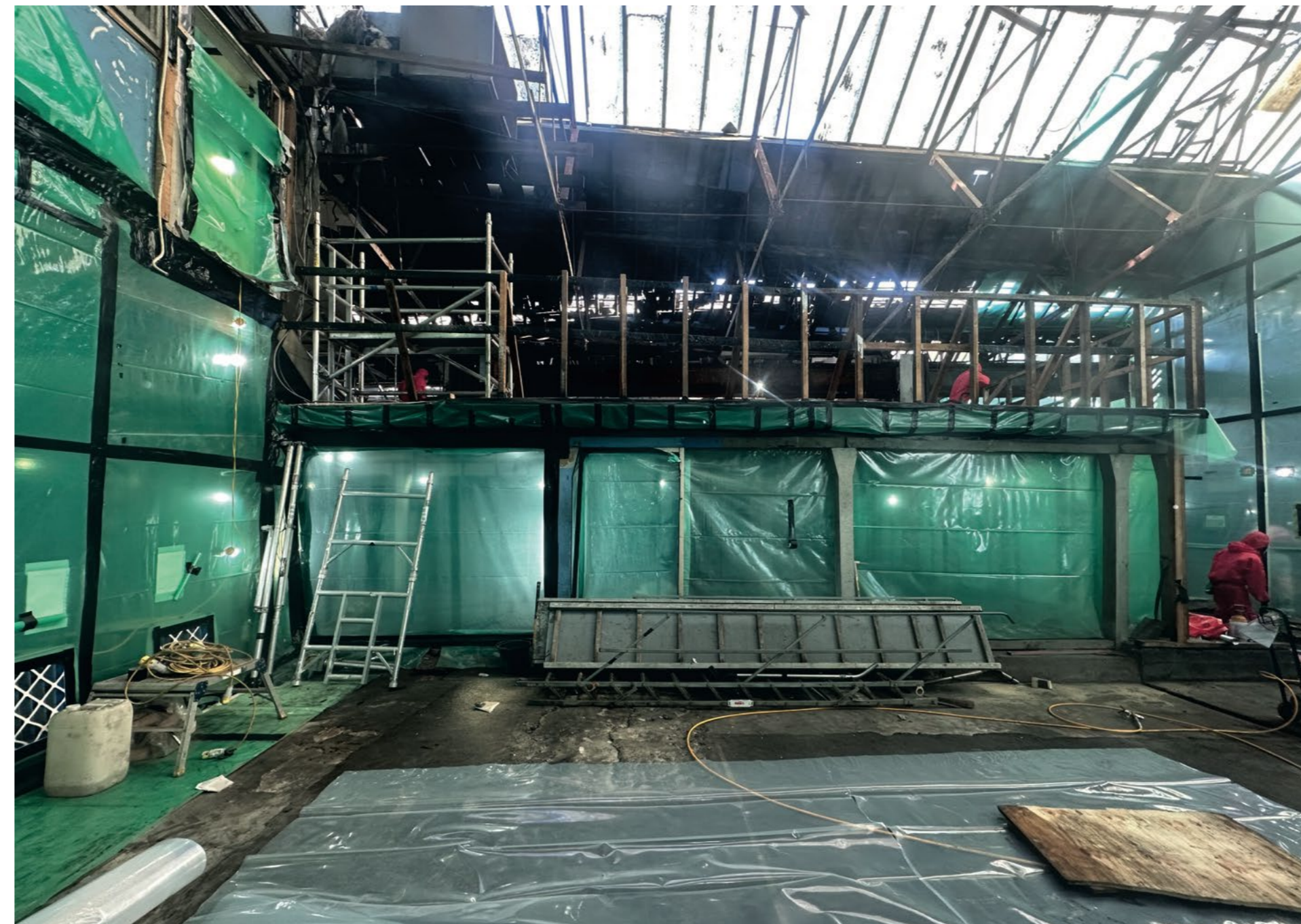
Machine Shop, asbestos removal
