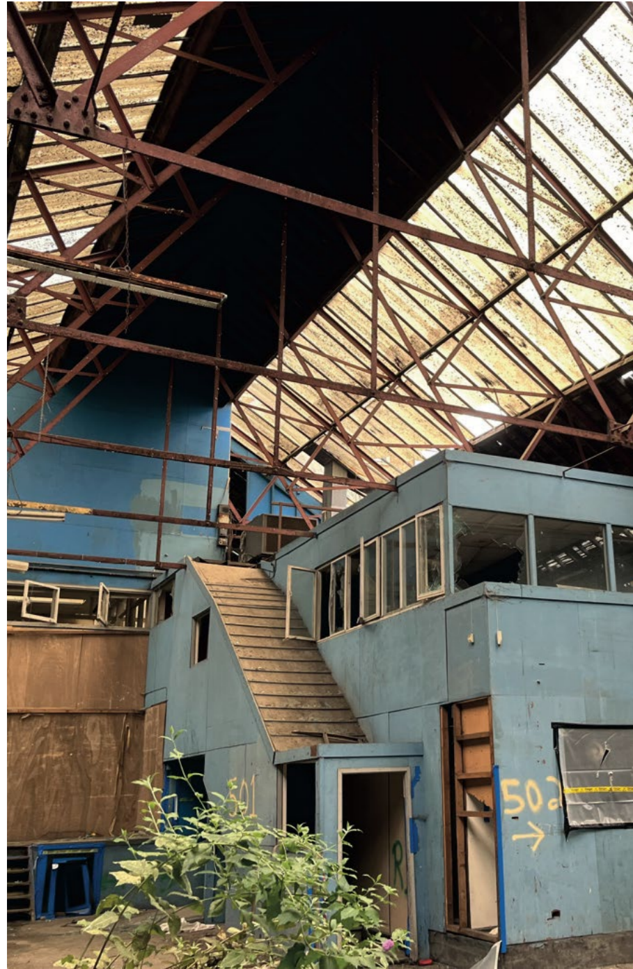
Machine Shop, modern additions
